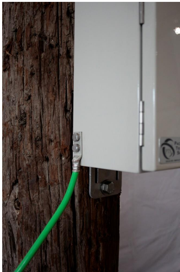
Figure 7: Example - Location of External Enclosure Ground Connection
