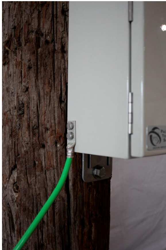
Figure 5: Mounting Location of External Enclosure Ground Connection
