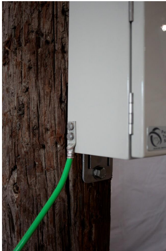
Figure 5: Mounting Location of External Enclosure Ground Connection
