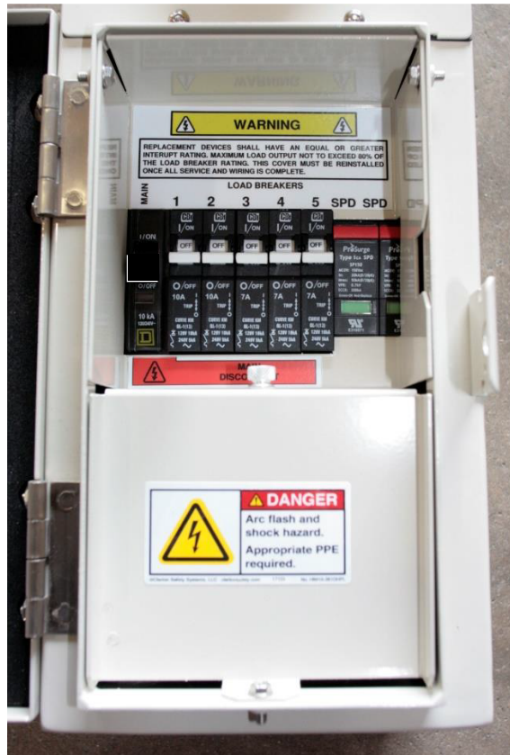
Figure 7: Dead Front Re-Installed
