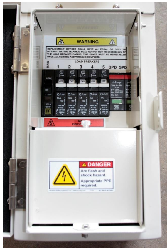
Figure 8: Dead Front Re-Installed
